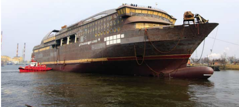
Partly equipped hull of Stavangerfjord launched at Gdansk.
